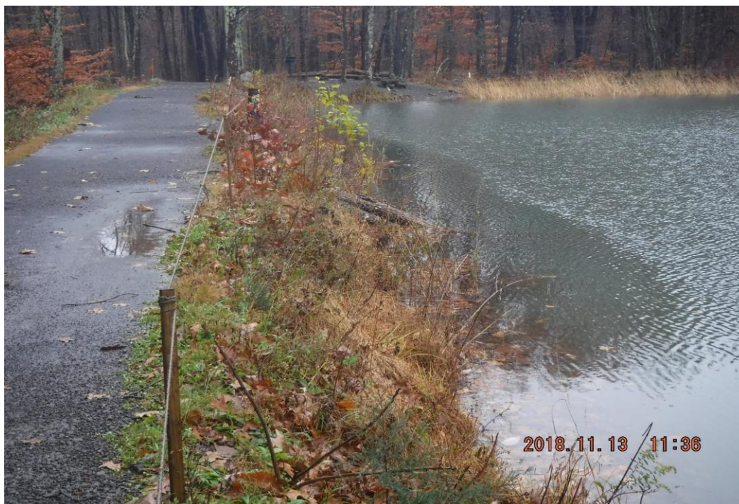
Photo 1 Dam ID# 193-5962 Duck Pond Dam 11/13/2018 Upstream slope View looking right from left end of dam
