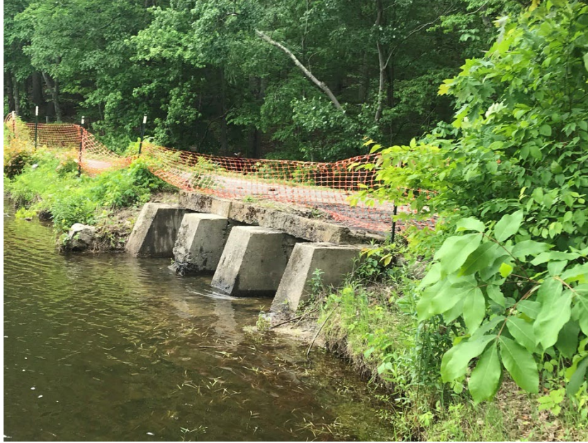
Figure 3-7 Duck Pond Dam spillway inlet
