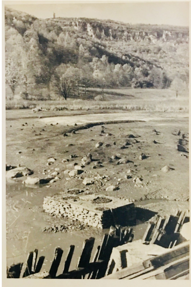
Figure 3-12 Low-level inlet structure (Mohonk archives, November 1932)
