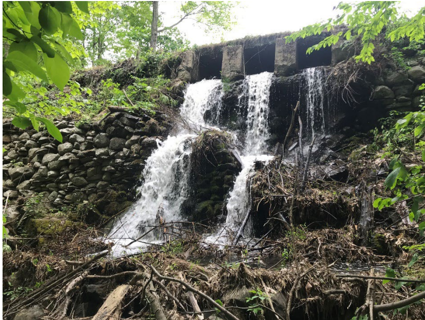
Figure 3-8 Downstream face of dam with spillway outlet (photo by SLR)
