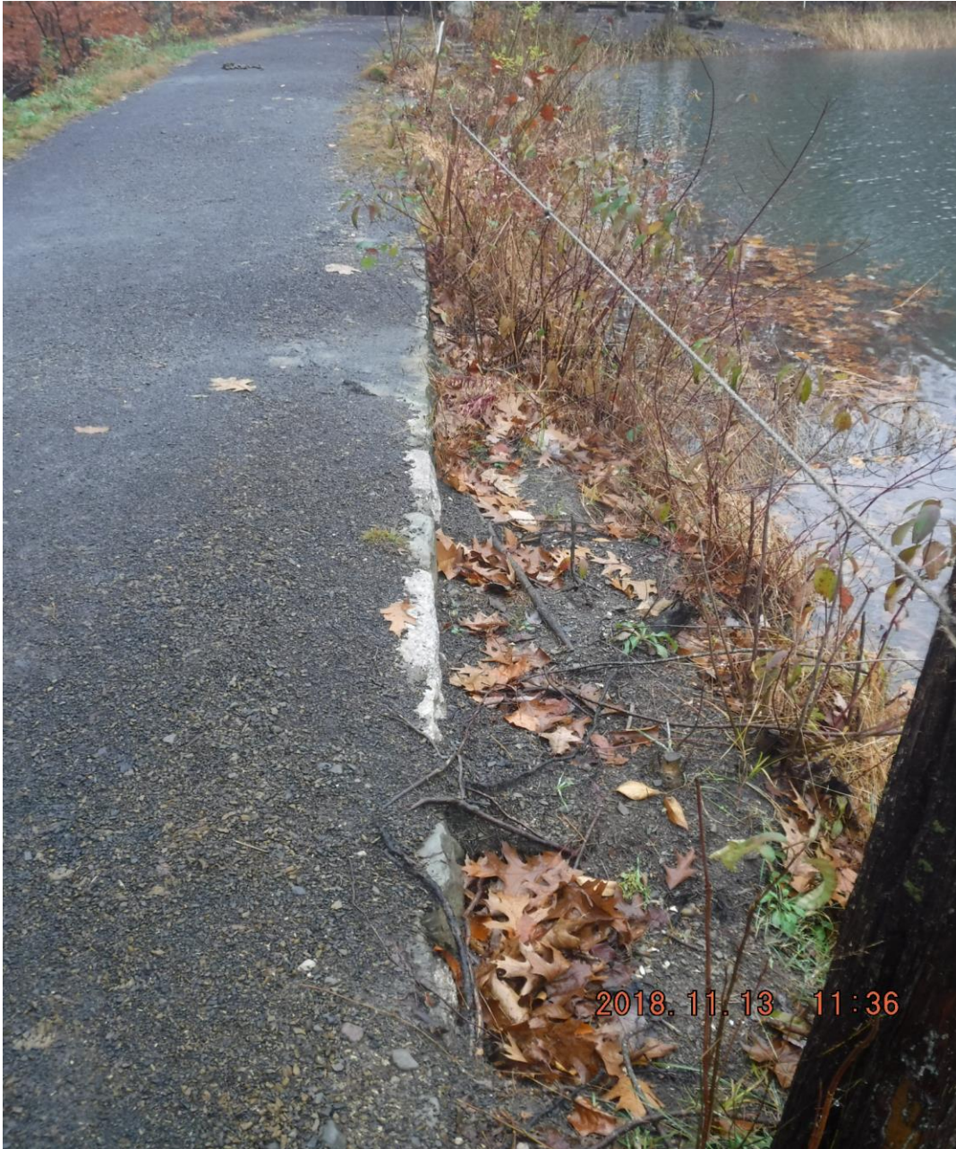
Photo 2 Dam ID# 193-5962 Duck Pond Dam 11/13/2018 Upstream crest/slope interface View looking right
