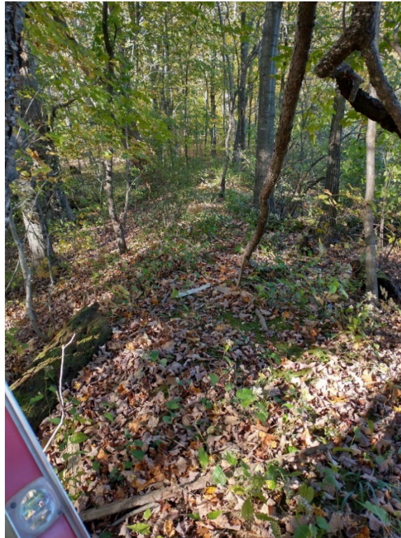
Figure 3-5 View along closure dike from seating area, looking west (photo by SLR)
