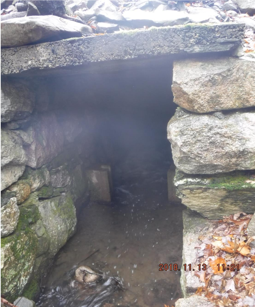
Photo 9 Dam ID# 193-5962 Duck Pond Dam 11/13/2018 Low level drain outlet
