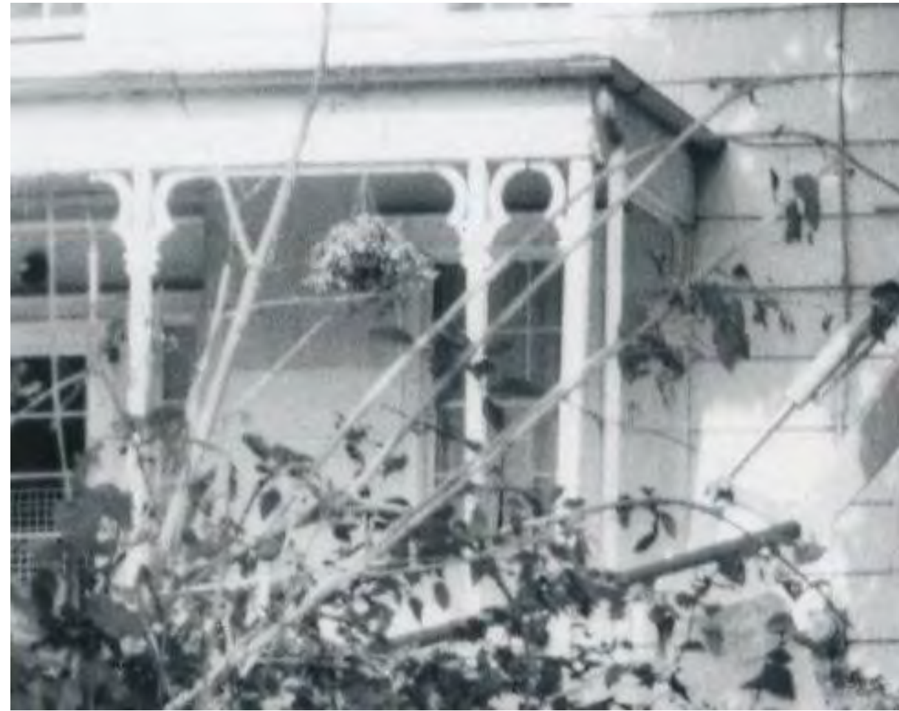
PHOTO OF ORIGINAL PORCH
