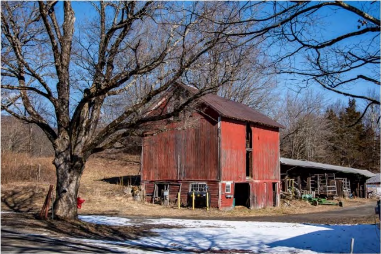
#B1-17 Brook Farm Barn 1 Southeast, 60 Gatehouse Road, New Paltz, NY 12561, 2/18/2024, Ulster
