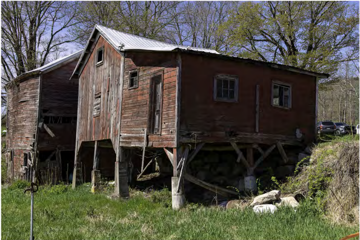
#B3-9 Brook Farm Barn 3 Northeast, 60 Gatehouse Road, New Paltz, NY 12561, 4/25/2024, Ulster
