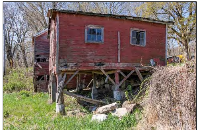
Fig. #74 Brook Farm Barn 3 Support Piers
