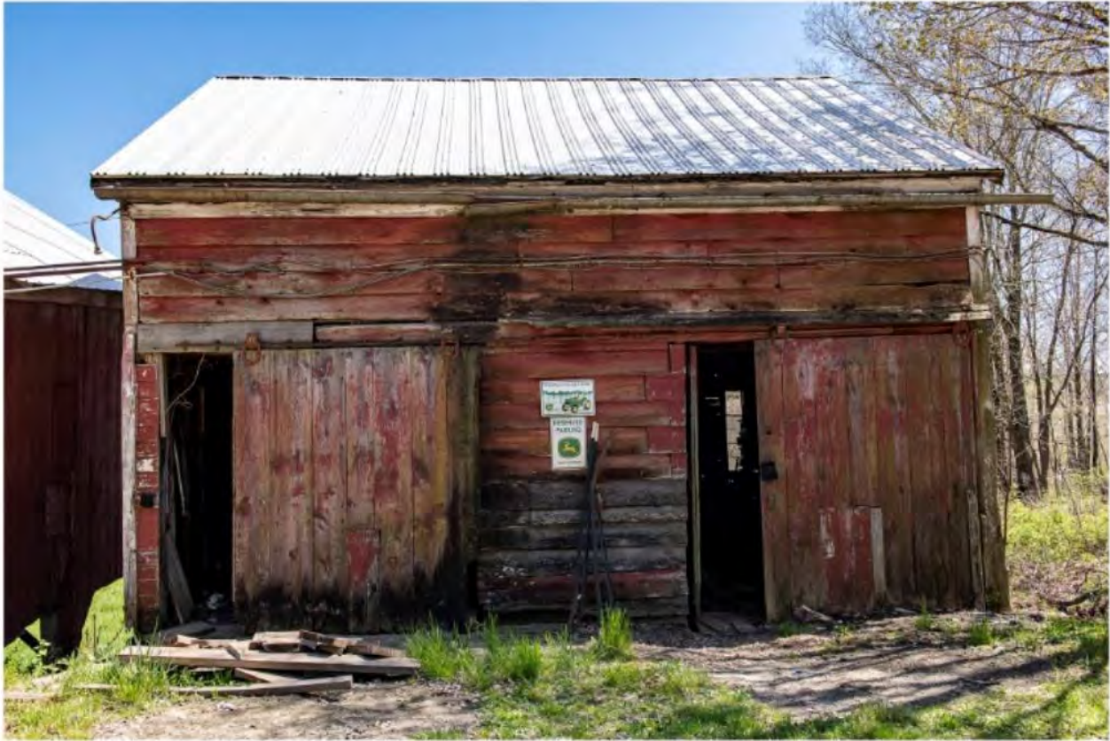
#B2-1 Brook Farm Barn 2 West, 60 Gatehouse Road, New Paltz, NY 12561, 4/26/2024, Ulster
