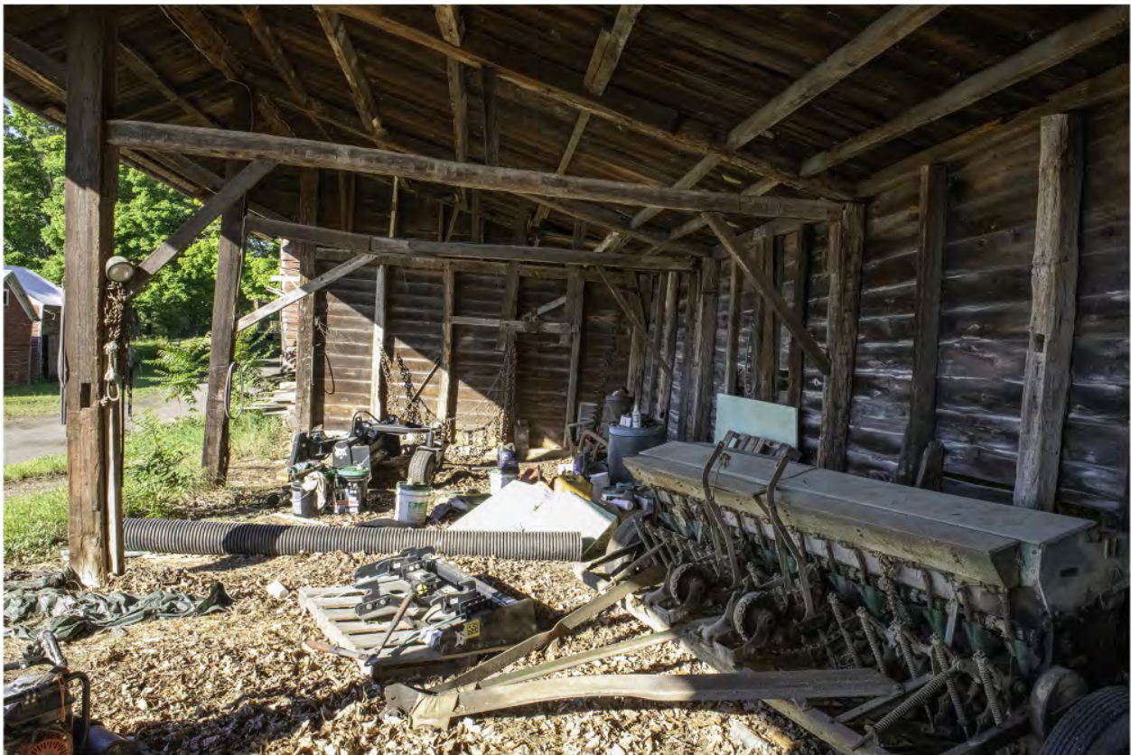
#OB-8 Brook Farm Outbuilding 1 Inside, 60 Gatehouse Road, New Paltz, NY 12561, 6/8/2024, Ulster
