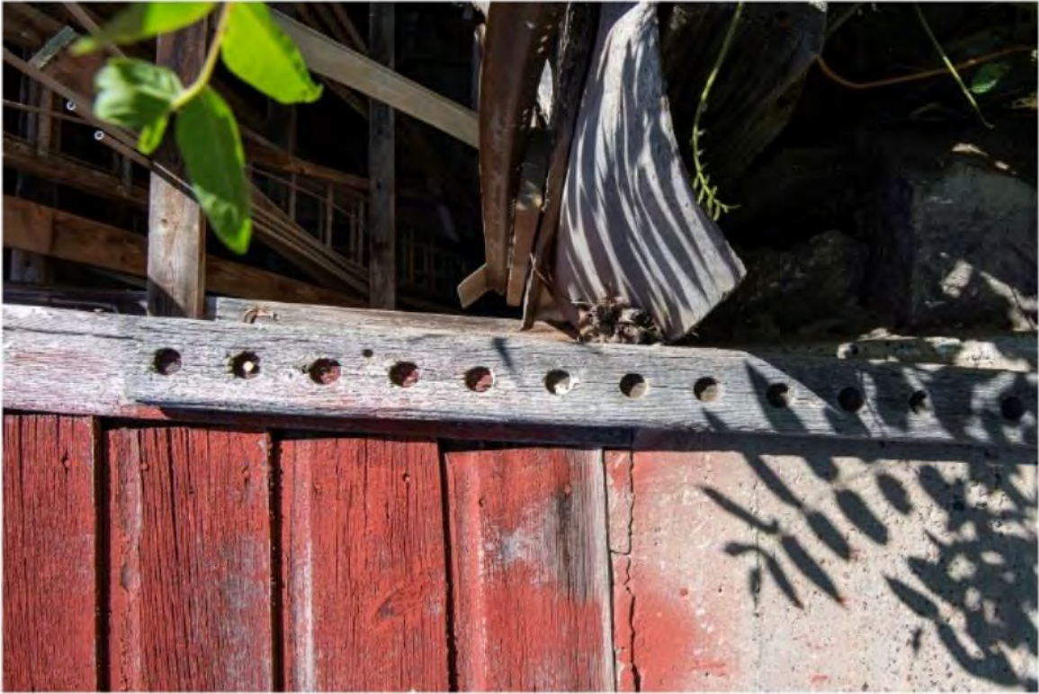
#B1-9 Brook Farm Barn 1 Northeast, 60 Gatehouse Road, New Paltz, NY 12561, 6/8/2024, Ulster
