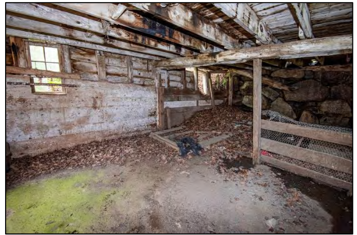
#51 Brook Farm Barn 2 Lower Level Stone Retaining Wall
