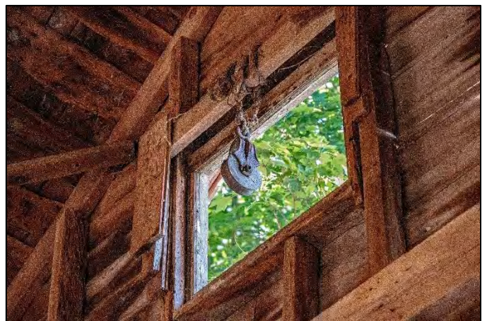
Fig. #32 Brook Farm Barn 1 north wall suspended pulley
