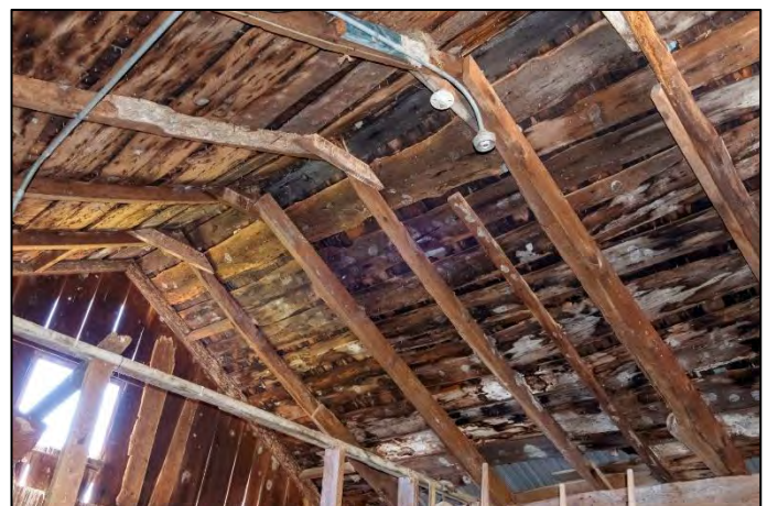
Fig. #86 Brook Farm Barn 3 Roof Cladding
