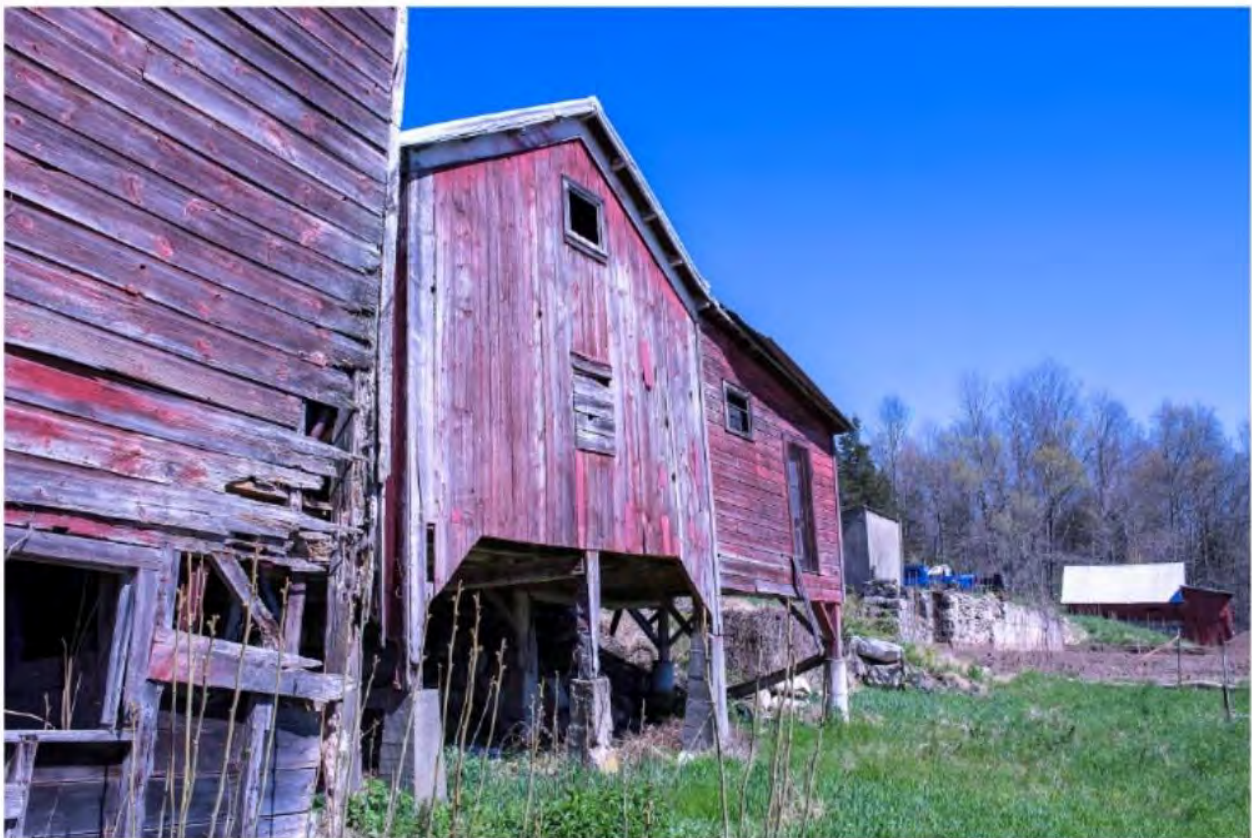
#B3-19 Brook Farm Barn 3 Southeast, 60 Gatehouse Road, New Paltz, NY 12561, 4/25/2024, Ulster
