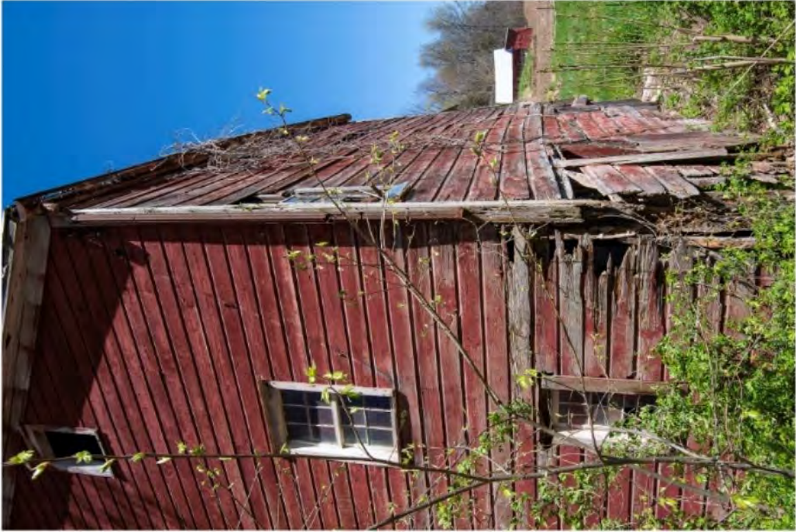
#B2-14 Brook Farm Barn 2 Southeast, 60 Gatehouse Road, New Paltz, NY 12561, 4/25/2024, Ulster
