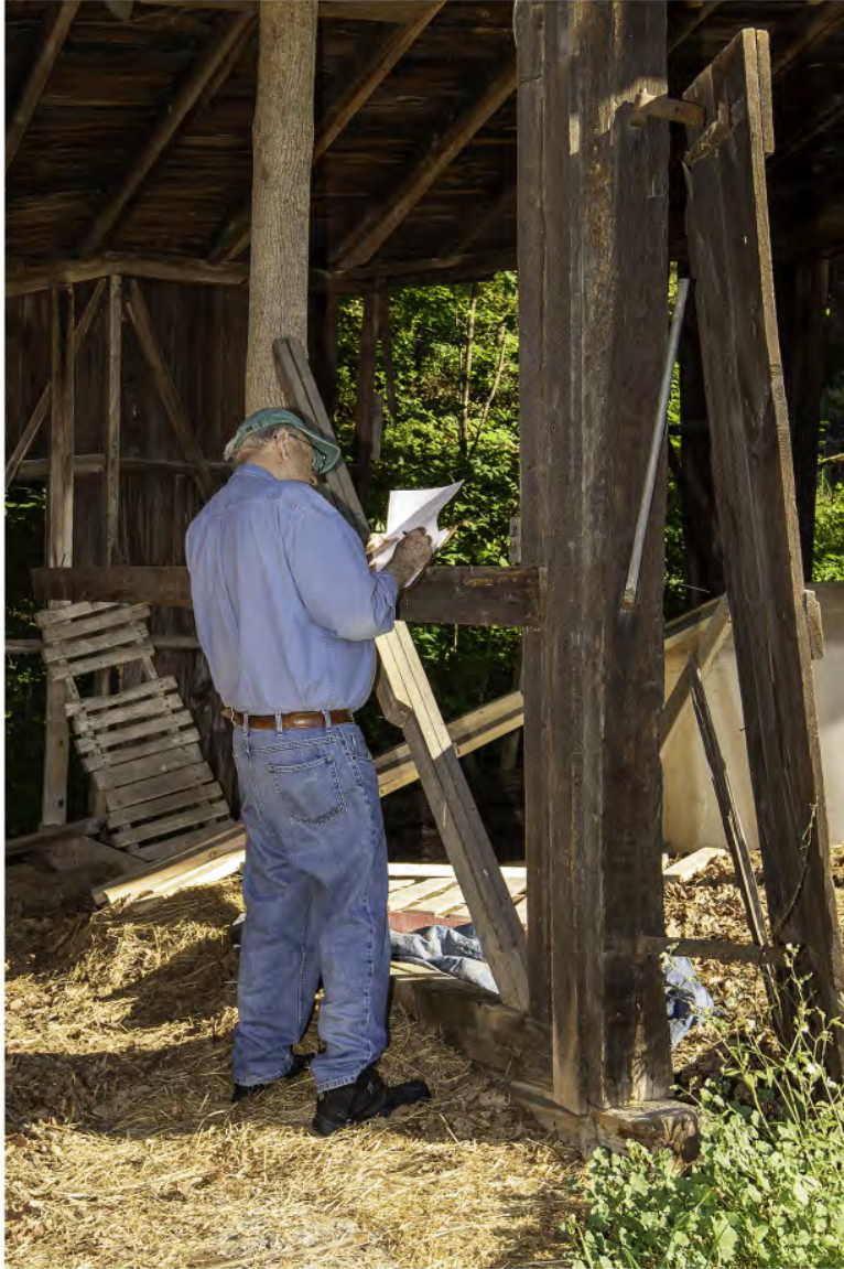
#OB-11 Brook Farm Outbuilding 1 Inside, 60 Gatehouse Road, New Paltz, NY 12561, 6/8/2024, Ulster
