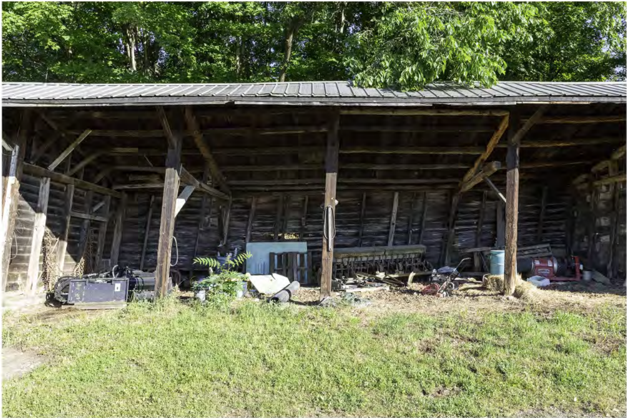
#OB-2 Brook Farm Outbuilding 1 East, 60 Gatehouse Road, New Paltz, NY 12561, 6/8/2024, Ulster
