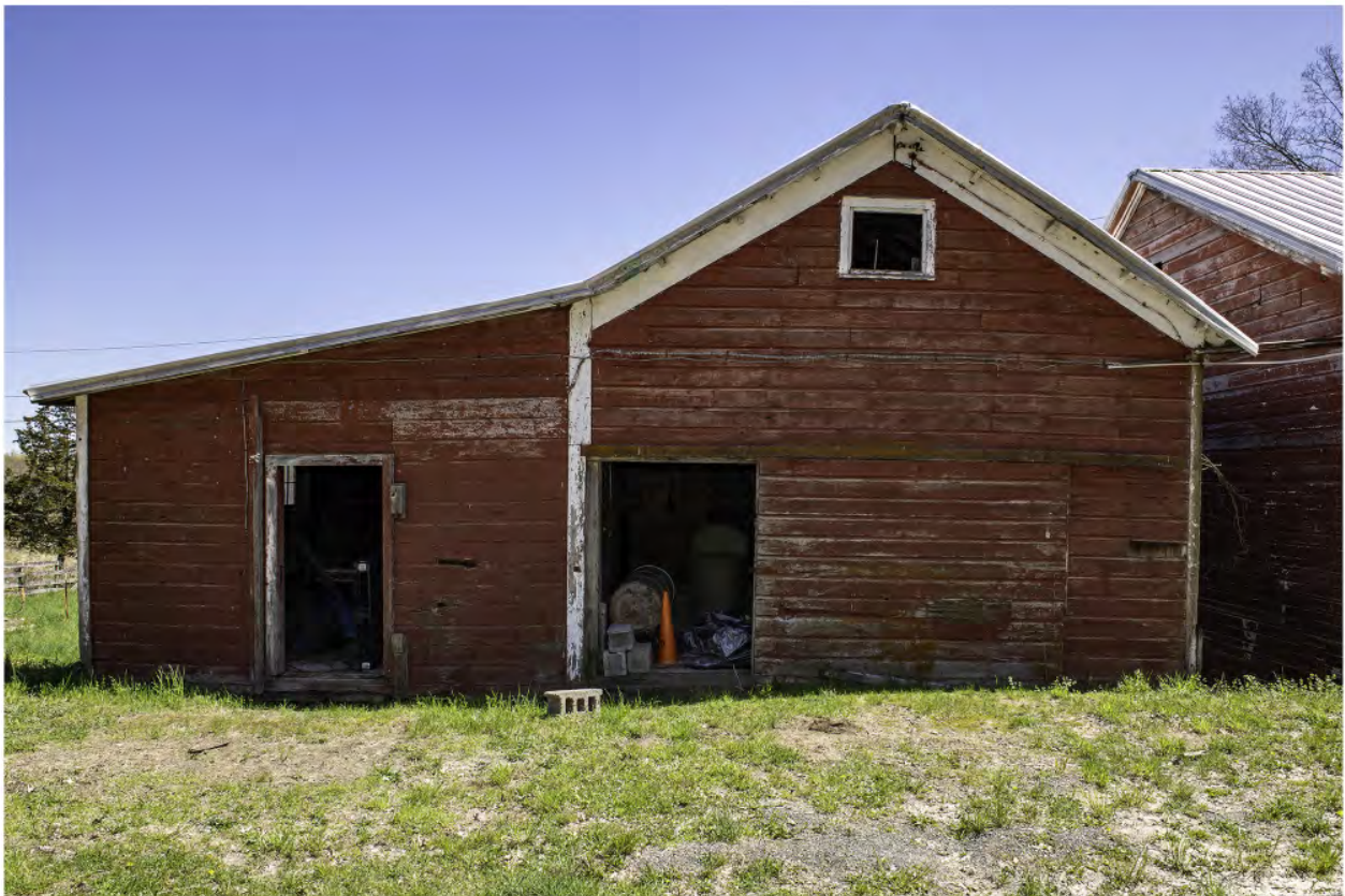
#B3-1 Brook Farm Barn 3 West, 60 Gatehouse Road, New Paltz, NY 12561, 4/26/2024, Ulster
