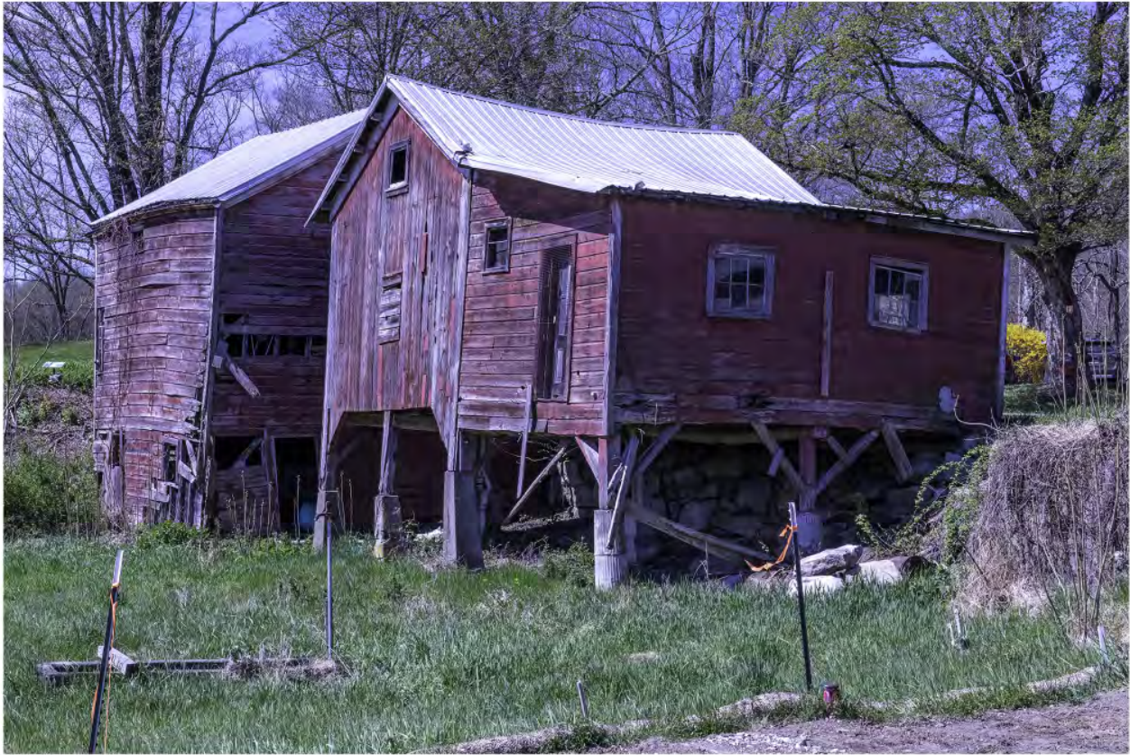
#B3-10 Brook Farm Barn 3 Northeast, 60 Gatehouse Road, New Paltz, NY 12561, 4/25/2024, Ulster
