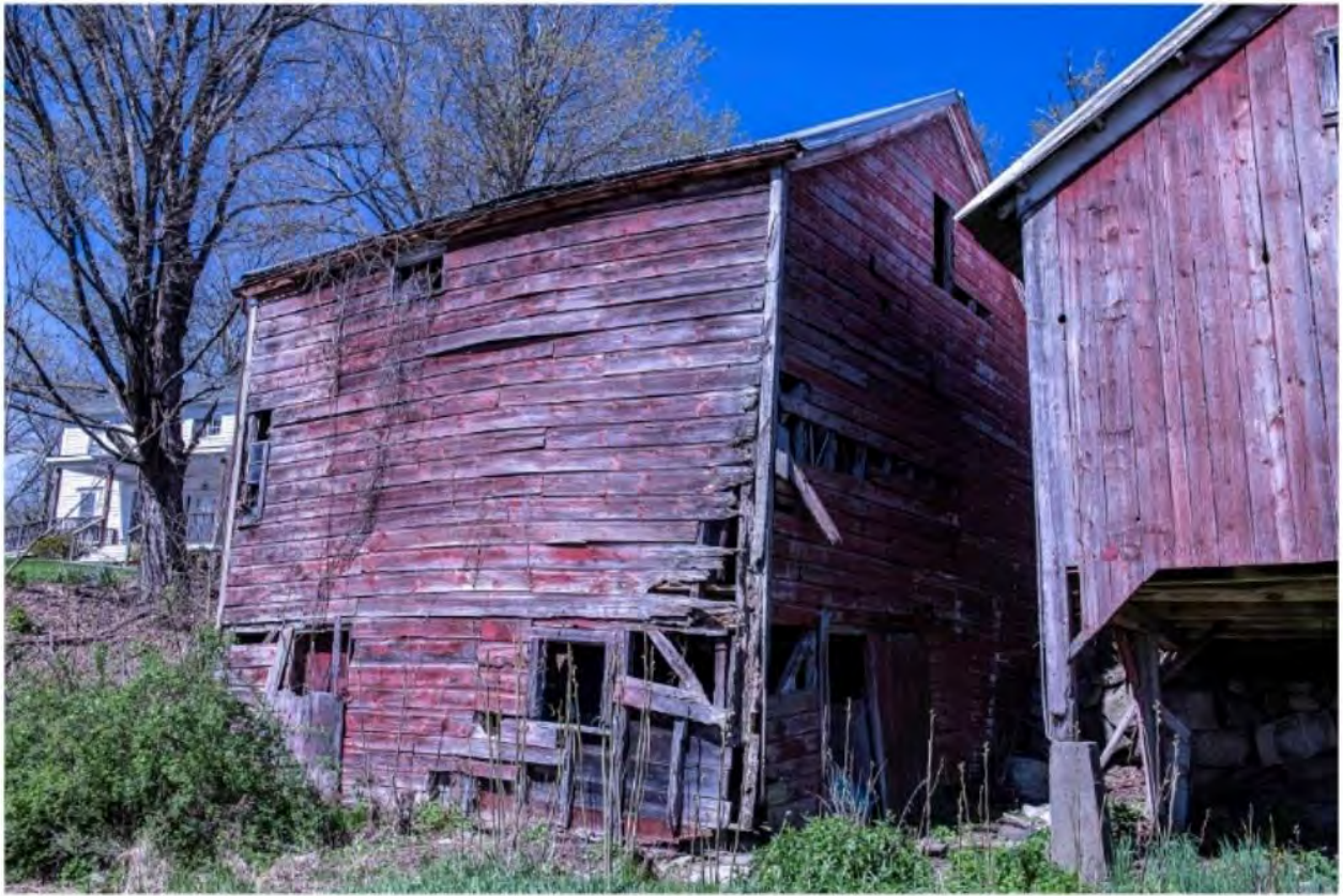
#B2-9 Brook Farm Barn 2 Northeast, 60 Gatehouse Road, New Paltz, NY 12561, 4/25/2024, Ulster
