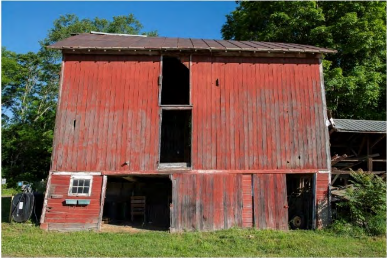
#B1-11 Brook Farm Barn 1 East, 60 Gatehouse Road, New Paltz, NY 12561, 6/8/2024, Ulster
