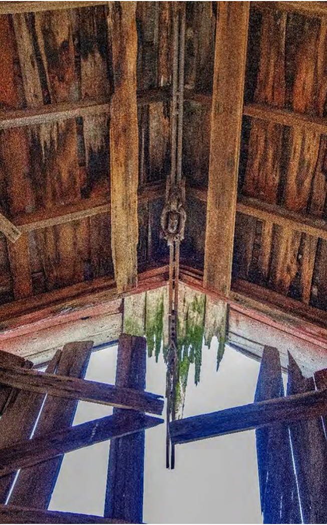
Fig. #27 Brook Farm Barn 1 hay carrier rail
