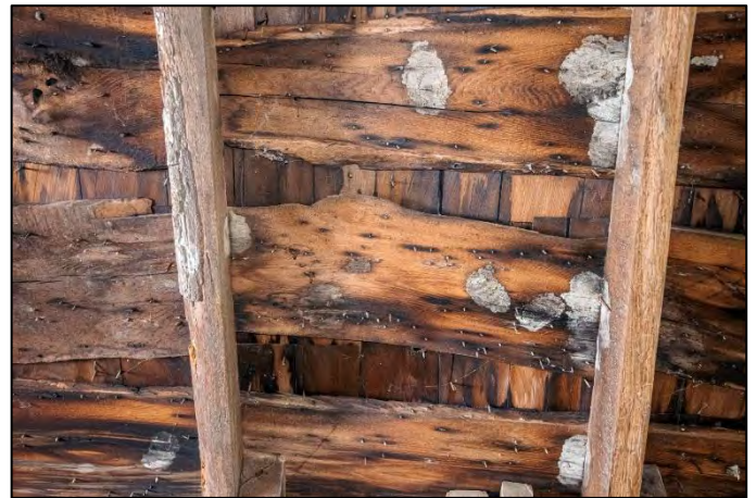
Fig. #69 Brook Farm Barn 2 Roof Cladding
