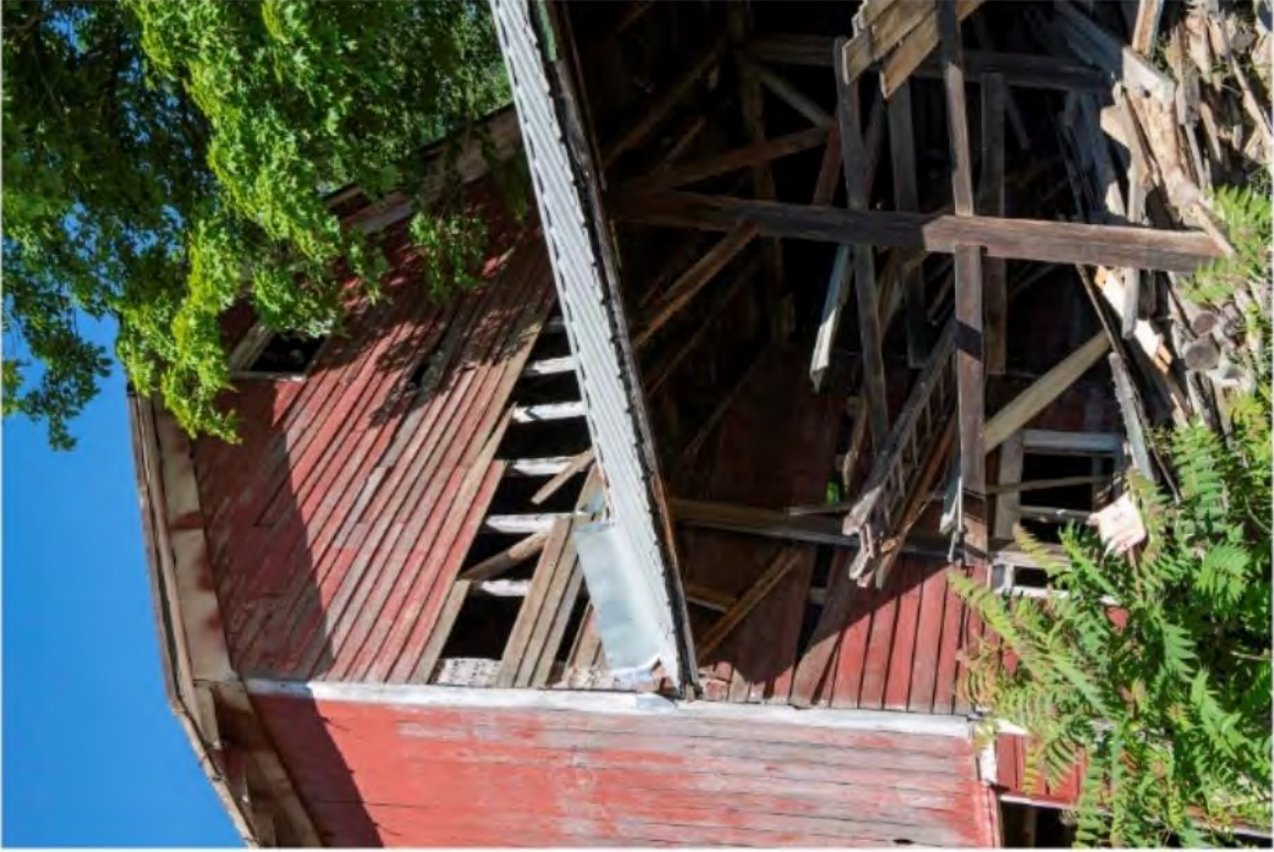
#B1-8 Brook Farm Barn 1 Northeast, 60 Gatehouse Road, New Paltz, NY 12561, 6/8/2024, Ulster
