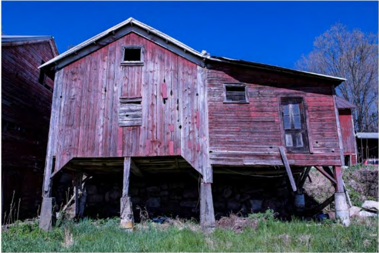
#B3-18 Brook Farm Barn 3 East, 60 Gatehouse Road, New Paltz, NY 12561, 4/25/2024, Ulster
