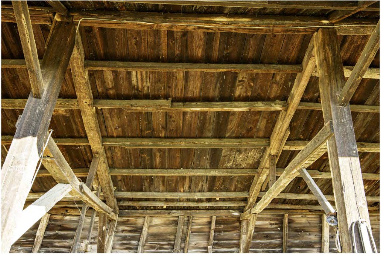
#OB-9 Brook Farm Outbuilding 1 Inside, 60 Gatehouse Road, New Paltz, NY 12561, 6/8/2024, Ulster
