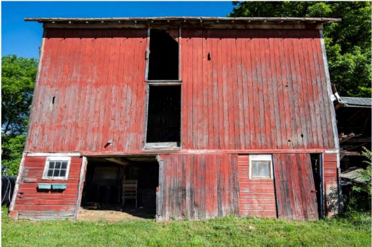
#B1-12 Brook Farm Barn 1 East, 60 Gatehouse Road, New Paltz, NY 12561, 6/8/2024, Ulster
