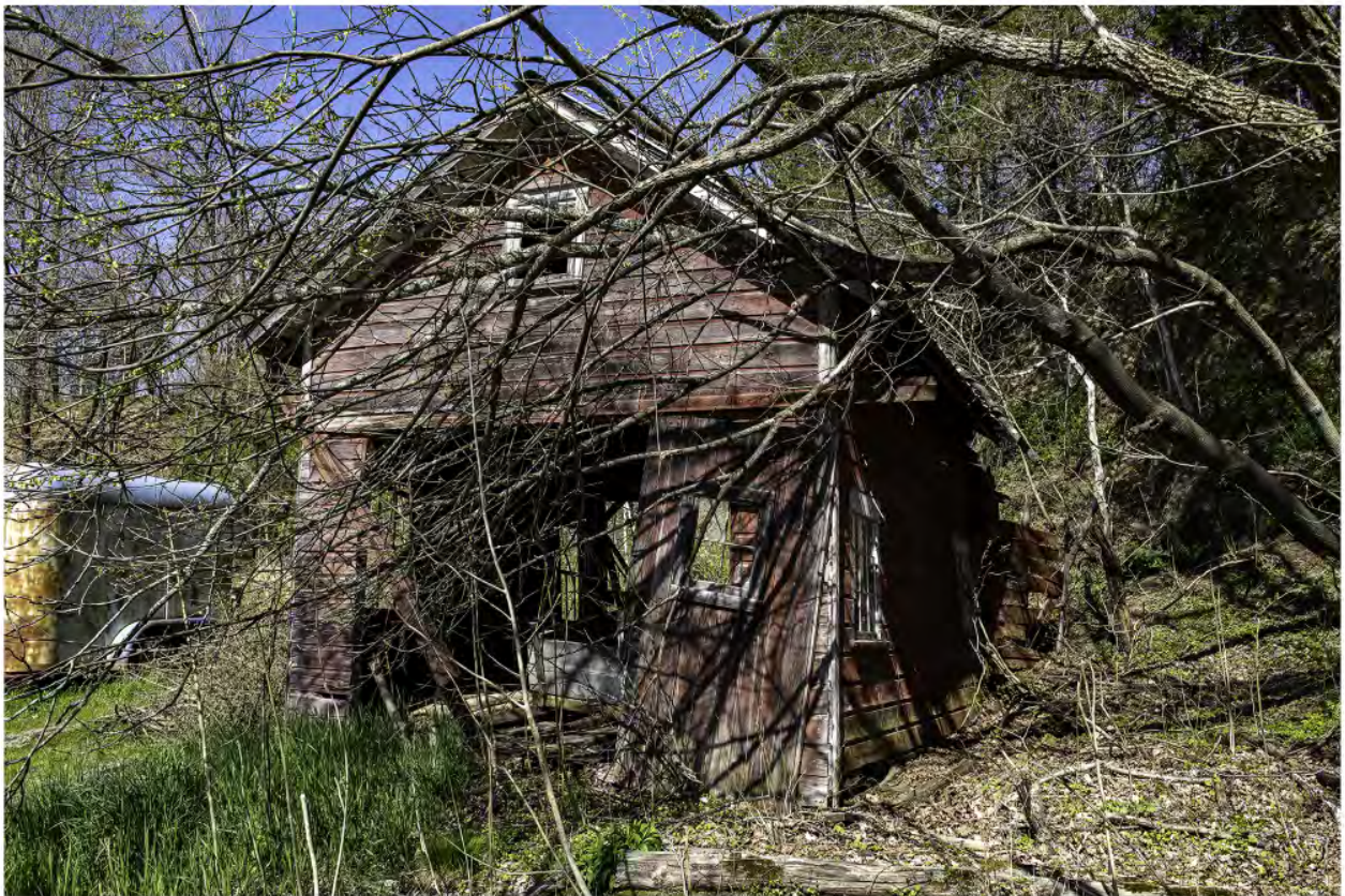
#B4-4 Brook Farm Barn 4 Northeast, 60 Gatehouse Road, New Paltz, NY 12561, 4/25/2024, Ulster
