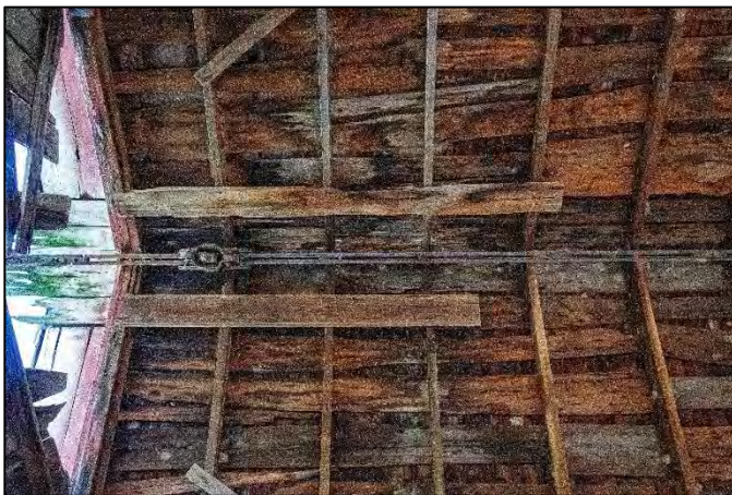
Fig. #28 Brook Farm Barn 1 hay carrier rail system
