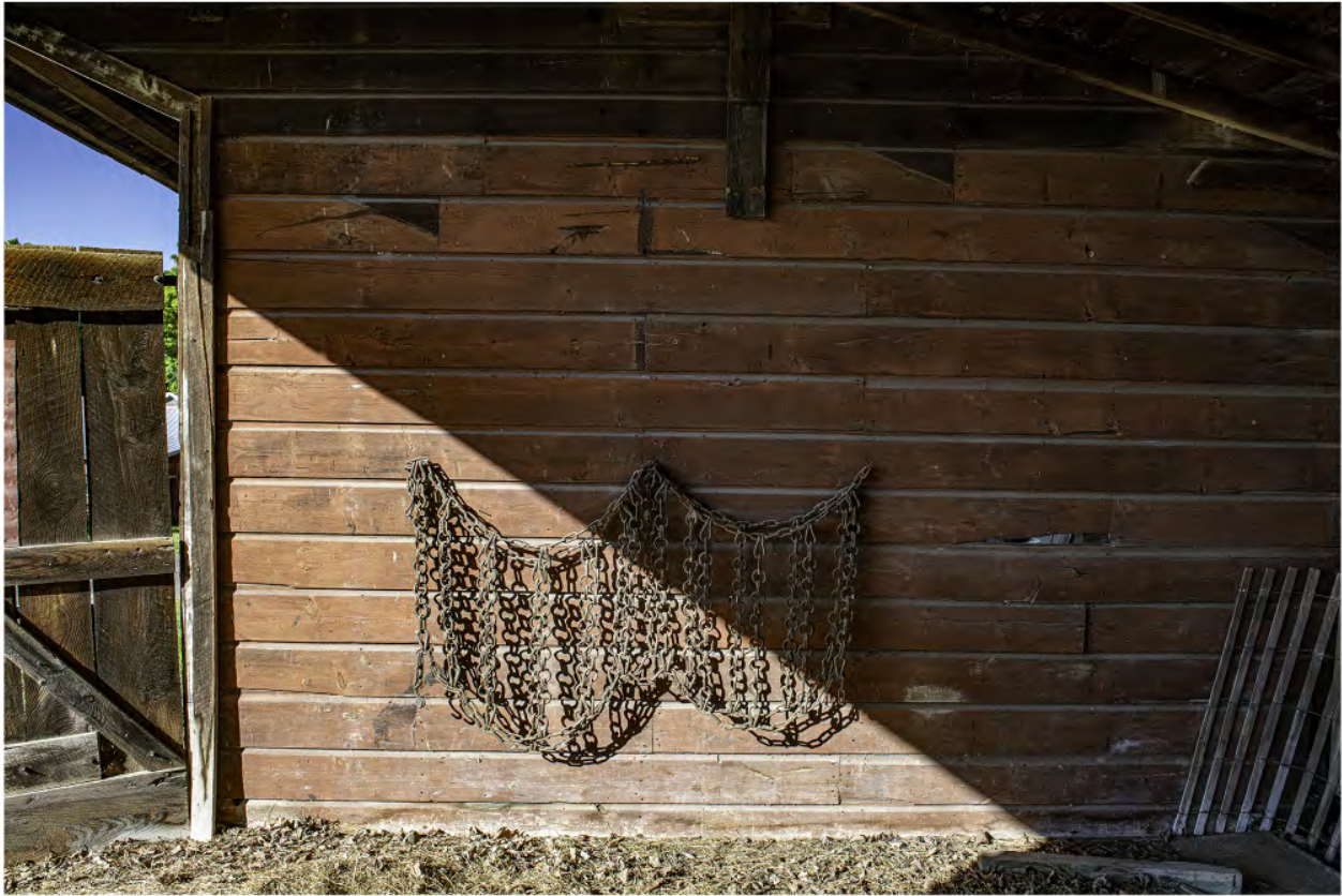
#OB-7 Brook Farm Outbuilding 1 Inside, 60 Gatehouse Road, New Paltz, NY 12561, 6/8/2024, Ulster
