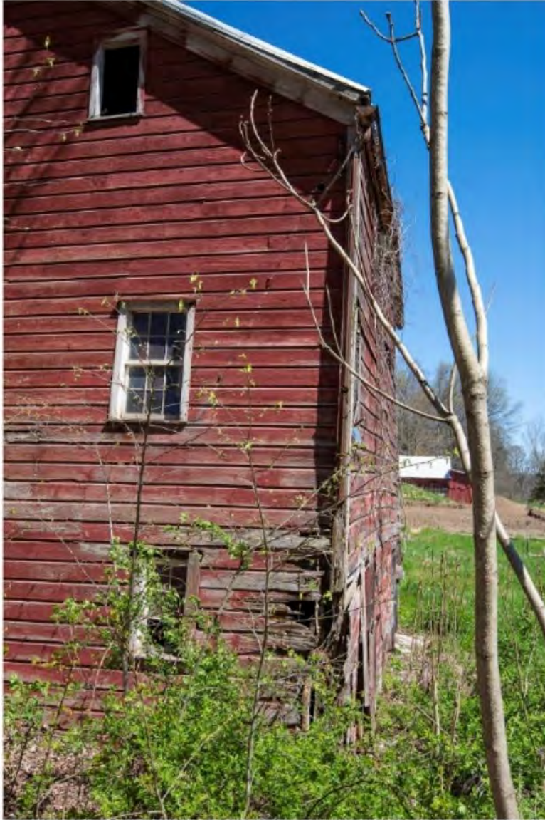
#B2-15 Brook Farm Barn 2 Southeast, 60 Gatehouse Road, New Paltz, NY 12561, 4/25/2024, Ulster
