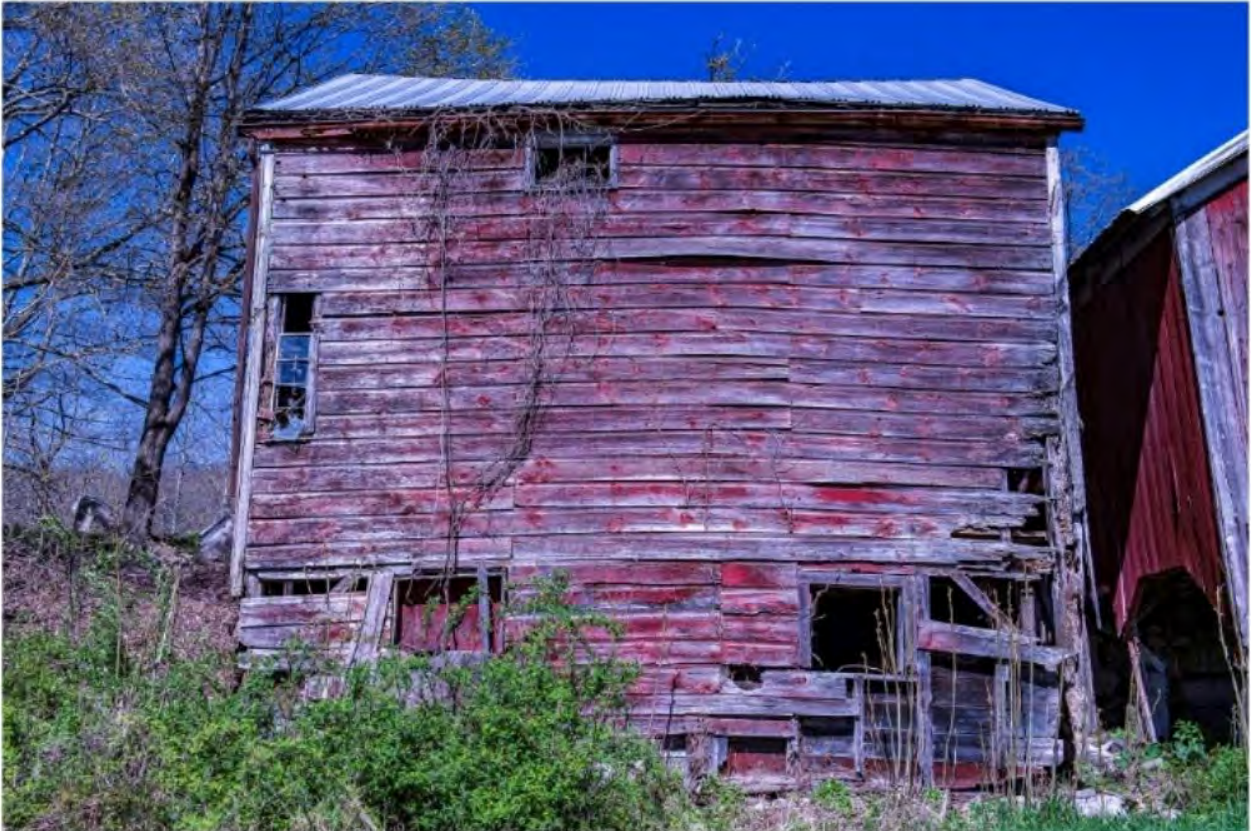
#B2-12 Brook Farm Barn 2 East, 60 Gatehouse Road, New Paltz, NY 12561, 4/25/2024, Ulster
