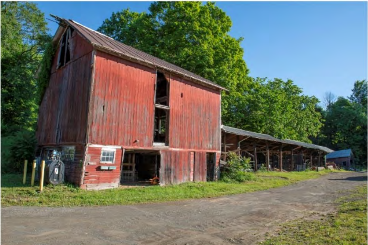
#B1-18 Brook Farm Barn 1 Southeast, 60 Gatehouse Road, New Paltz, NY 12561, 6/8/2024, Ulster
