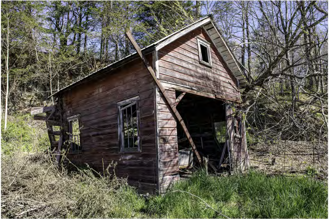
#B4-5 Brook Farm Barn 4 Southeast, 60 Gatehouse Road, New Paltz, NY 12561, 4/25/2024, Ulster
