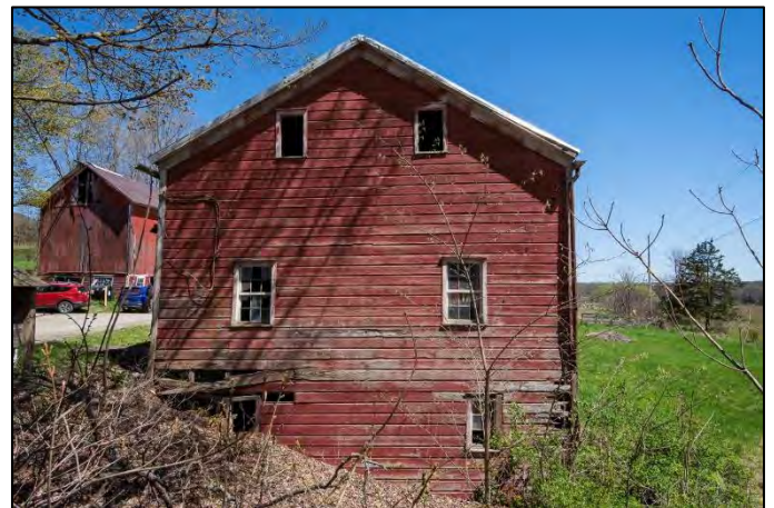
Fig. #67 Brook Farm Barn 2 Six over Six Windows
