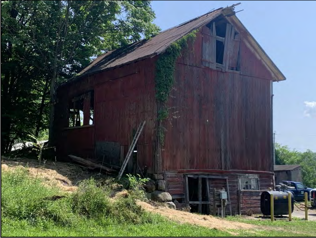
Photo 1-Barn 1: Overall exterior view of Barn 1.
