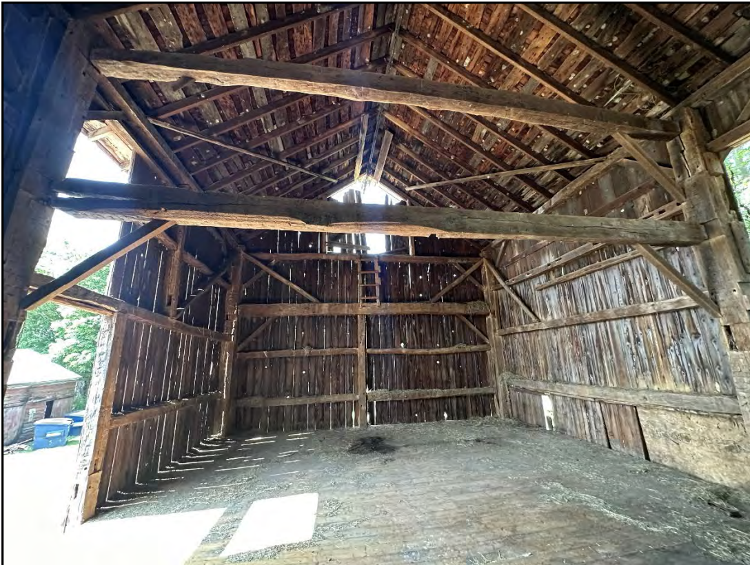
Photo 2-Barn 1: View of Southern and middle bents.
