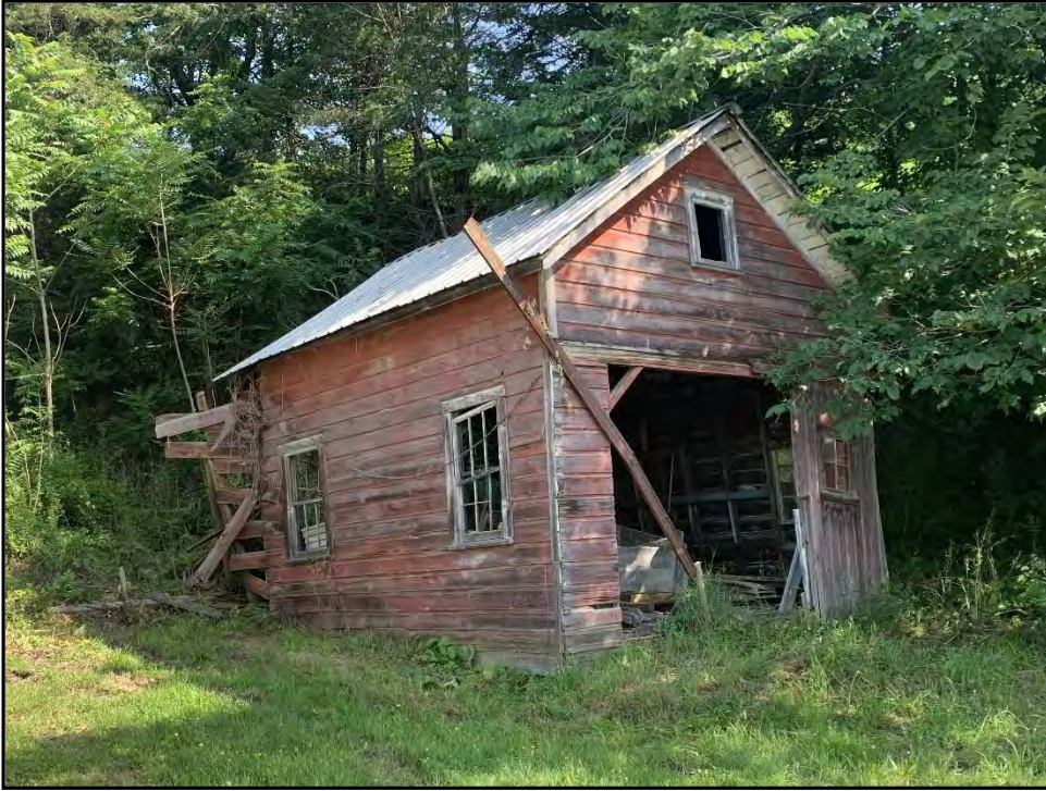
Photo 23-Barn 4: Overall view of Barn 4.
